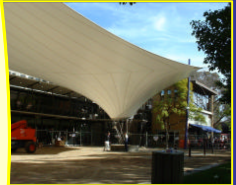
University of Melbourne, Victoria Membrane fabrication and installation for Tecraft
